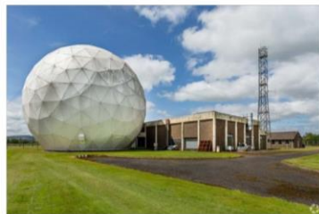
External image of existing Building
